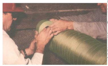
REFRASIL Irish slit tape is spiral wrapped around water cooled skid pipe in steel mill slab reheat furnace, securing REFRASIL RB1800 blanket insulation, providing protection in environments up to 2300°F.
